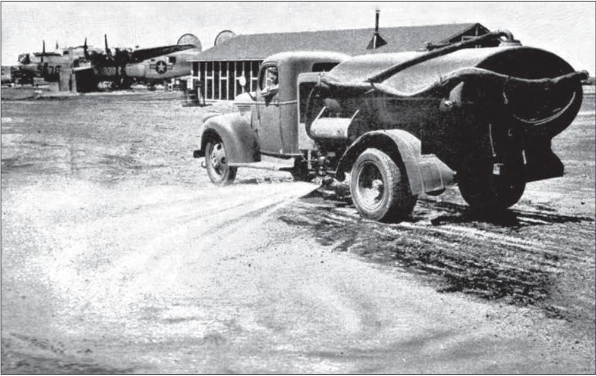
U.S. Army troops water an air installation in 1945 to reduce dust and erosion. They followed the water application with a layer of oil. U.S. War Department Technical Manual TM 5-630.
