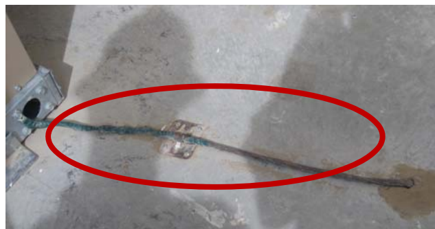
Figure 2. Exposed Ground Wires Put Personnel and Equipment at Risk
