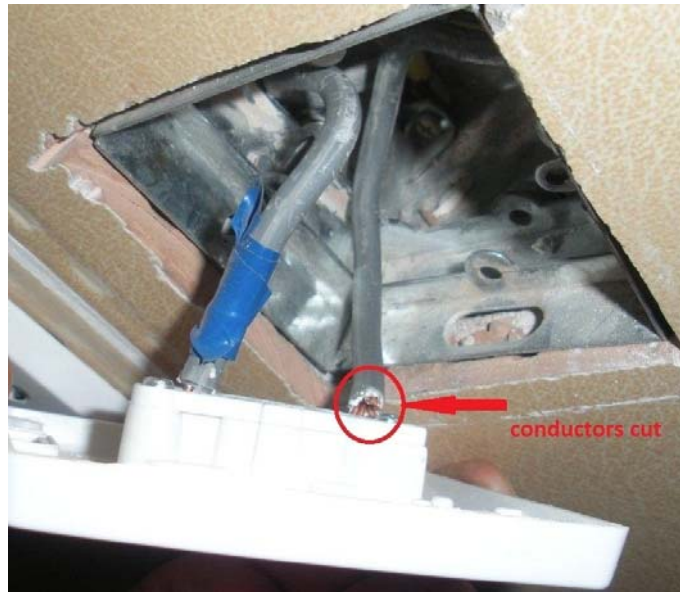
Figure 3. Cutting Strands of Wire Results in a Fire Hazard
