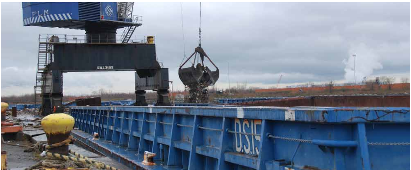
Debris from Hurricane Sandy loaded onto barges. (Photo courtesy of USACE-CW)
