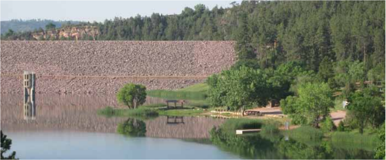
Rainfall in early July brought the pool elevation at Cold Brook reservoir to an elevation of 3585.0 feet, which is slightly above the top of the conservation pool level. (Photo by Paula Andrie)
