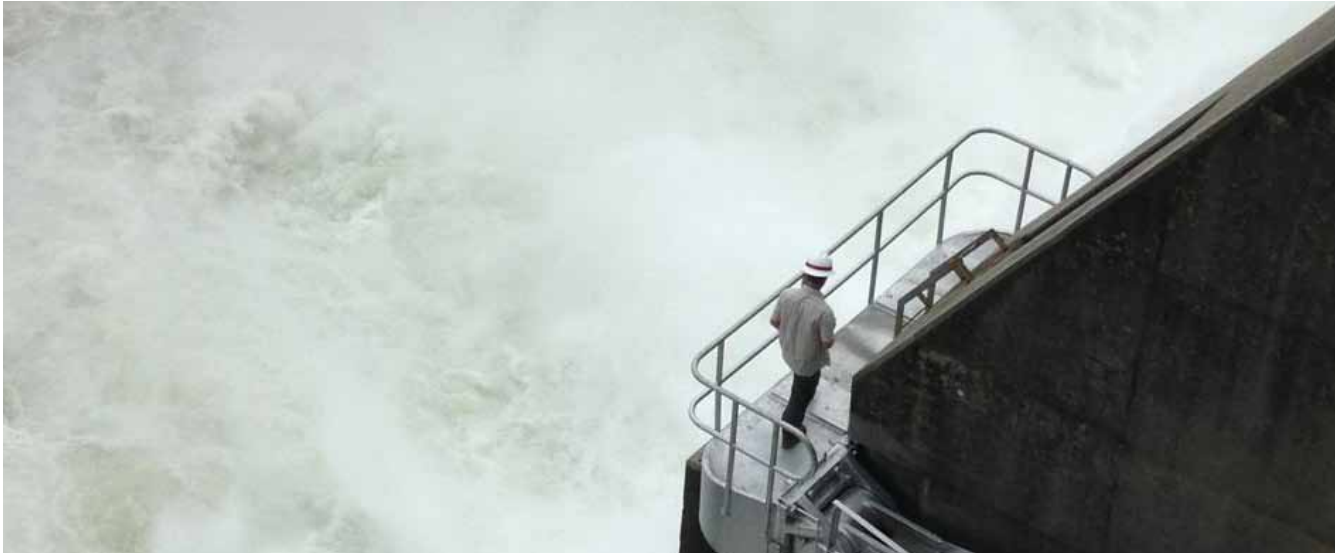
The U.S. Army Corps of Engineers Savannah District test the spillway gates at the J. Strom Thurmond Dam to ensure the gates can be activated properly in the event of an emergency. (USACE-CW photo by Billy Birdwell)
