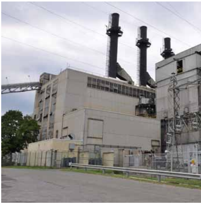
Goddard Power Plant, the last coal-fired power facility operated by the Navy, will be demolished and replaced by a natural-gas cogeneration facility and infrastructure that will provide steam critical to energetic mission activities as well as 3.5 megawatts of electricity. (U.S. Navy photo by Gary Wagner/Released)
