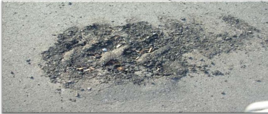
Figure 3. Asphalt Beginning to Deteriorate (NOSC Exterior Parking Lot)
