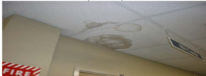
Figure 2. Residue From Roof Leaks (NOSC Office)
