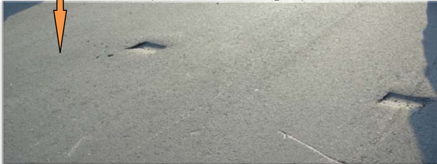
Figure 5. Asphalt After a Vehicle Has Been Parked (NOSC Exterior Parking Lot)
