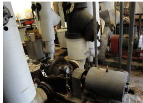
Two-pipe HVAC system in building SC-1 of the Joint Forces Staff College, Naval Support Activity, Norfolk, Virginia. Photo taken by DoD Office of Inspector General
