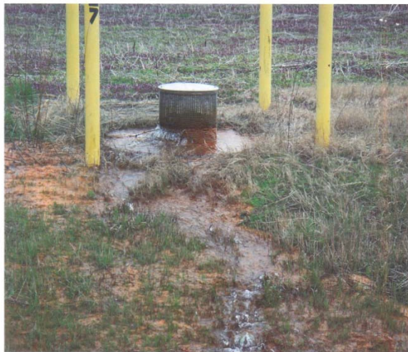
Figure 2. St. Francis River Basin Relief Well
