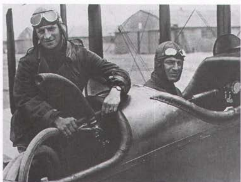
The de Havilland DH-4B tanker dangles a hose for the DH-4B receiver to grab over Rockwell Field (top). In the tanker, 1st Lt. Frank W. Seifert holds the hose in the rear cockpit while the pilot, 1st Lt. Virgil Hine, is in the front (left). Capt. Lowell H. Smith flew the receiver, and 1st Lt. John P. Richter handled the hose (bottom).
