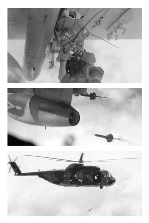
**Sensors**. A seismic sensor is attached to a pylon on a Navy OP–2E (top), an OP–2E releases a sensor (center), and a CH–3 releases a seismic sensor (bottom).
