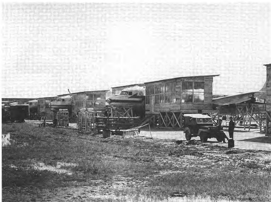
"The 200-hour inspection was more than a casual evaluation." C-54s in the wooden inspection docks constructed at Oberpfaffenhofen air depot, Oberpfaffenhofen, Germany. ( U.S. Air Force. )
