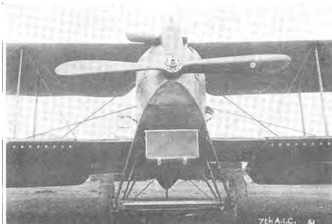
Loaded bomb rack on a Breguet.
