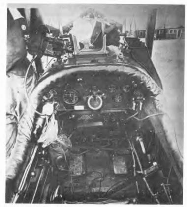
Radio set installed in a DH-4.
