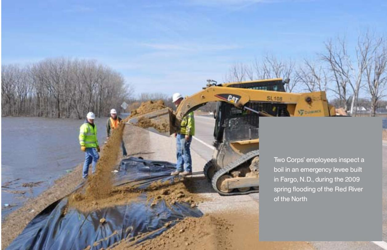
Two Corps' employees inspect a boil in an emergency levee built in Fargo, N.D., during the 2009 spring flooding of the Red River of the North
