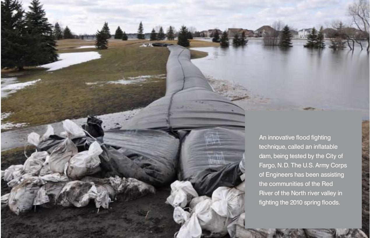
An innovative flood fighting technique, called an inflatable dam, being tested by the City of Fargo, N.D. The U.S. Army Corps of Engineers has been assisting the communities of the Red River of the North river valley in fighting the 2010 spring floods.
