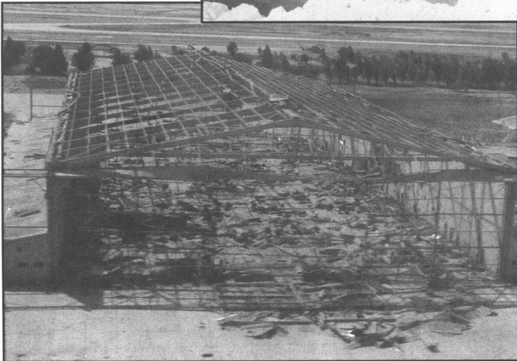
BOTTOM: A Matter of Interpretation—a target at Talil Air Base, Iraq, categorized as “moderately” damaged by intelligence analysts. The air planners considered it destroyed.
