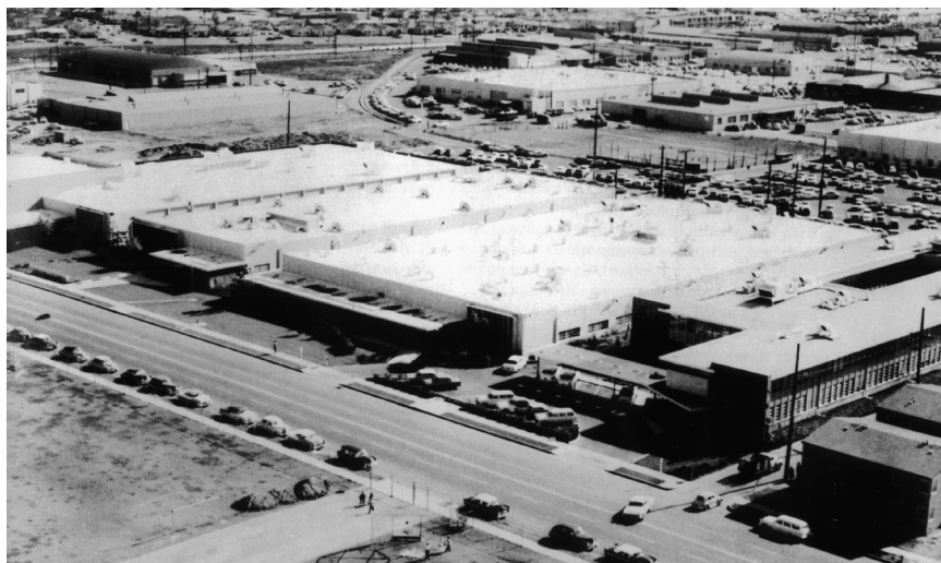
Buildings used by the Space Technology Laboratories, the successor to R-W’s Guided Missile Research Division, in July 1959.
