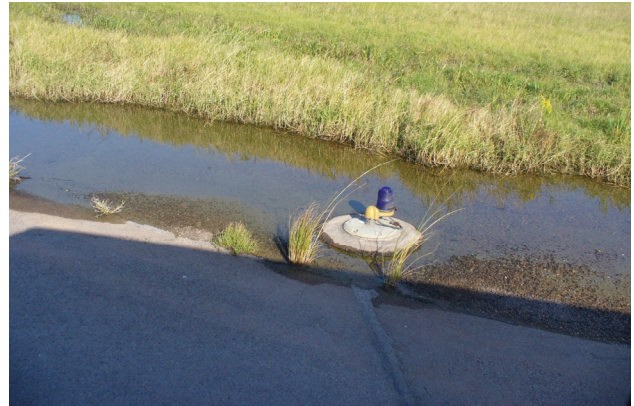
Poor Drainage Along Runways at NAS/JRB New Orleans
