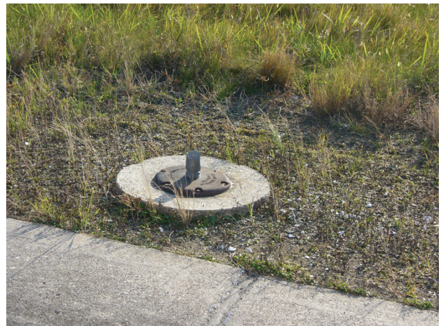
Missing Runway Lights at NAS/JRB New Orleans
