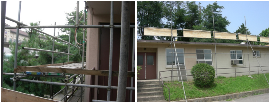
Figure 1. Scaffolding Around a Building Figure 2. Fall Protection for Roof Work
