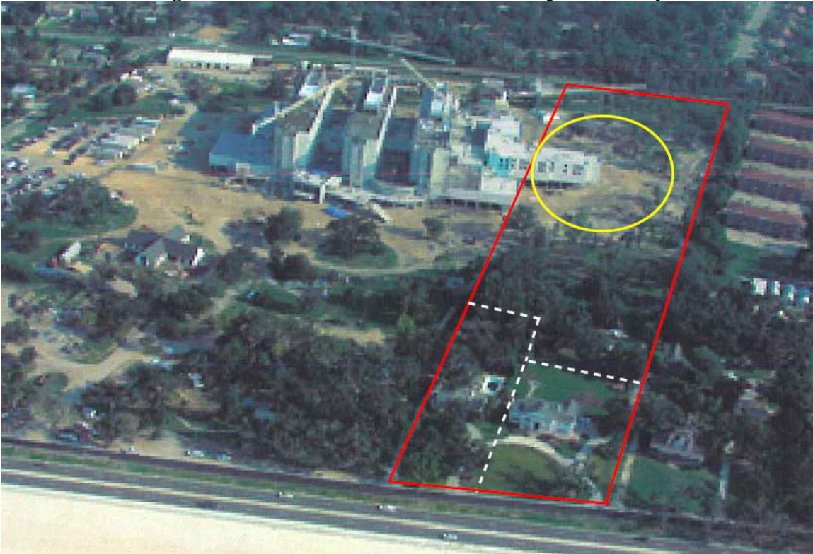
Figure 1. Aerial View of the AFRH-Gulfport Facility
