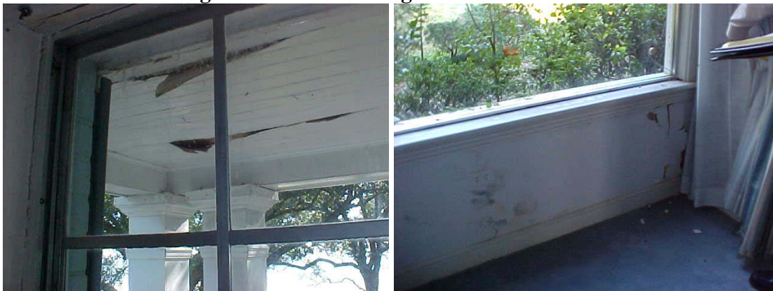
Figures 4 and 5. Damage to Beachfront Homes
