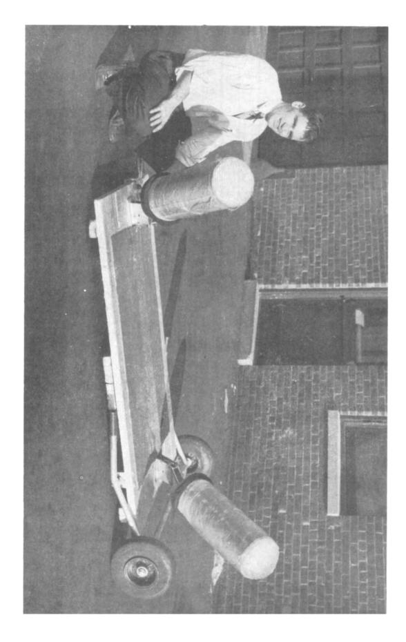
Figure 24 General Mills launching platform for large balloons.
