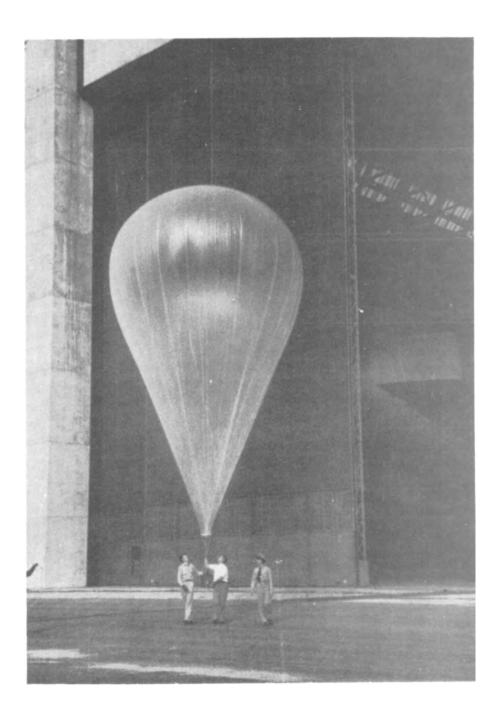
Figure 2 Teardrop, .001" polyethylene balloon, 20 foot in diameter, designed by General Mills, Inc.
