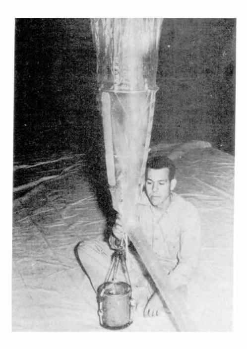
Figure 5 Two foot appendix, stiffened, shown on a General Mills ballon. The swollen inflation tube indicates that the balloon is being filled.
