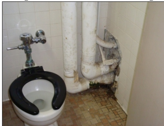
Figure 4. Deteriorated Plumbing
