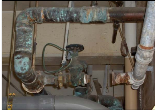
Figure 3. Deteriorated Heating, Ventilation, and Air Conditioning System
