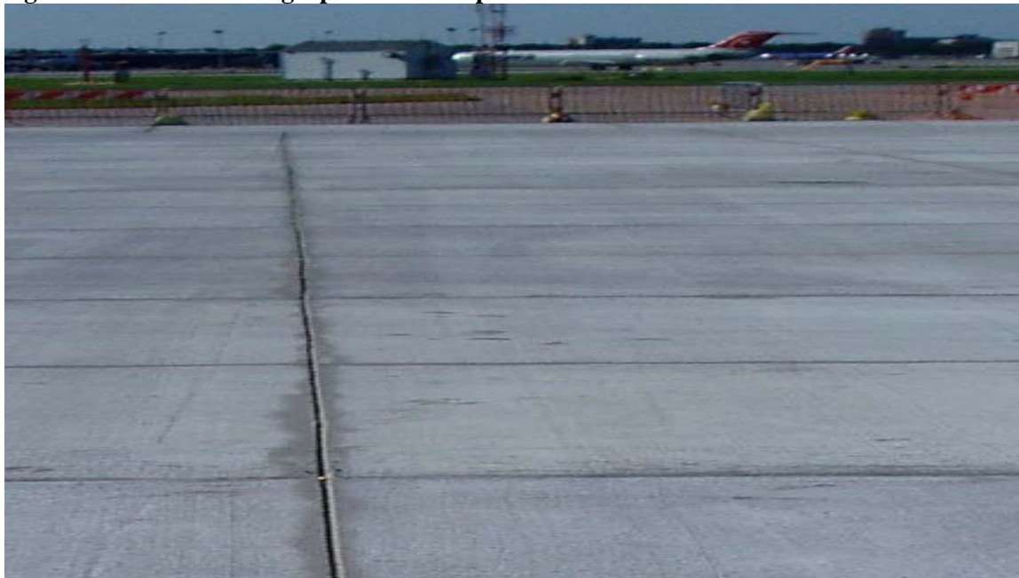
Figure 3. Aircraft Parking Apron After Repairs
