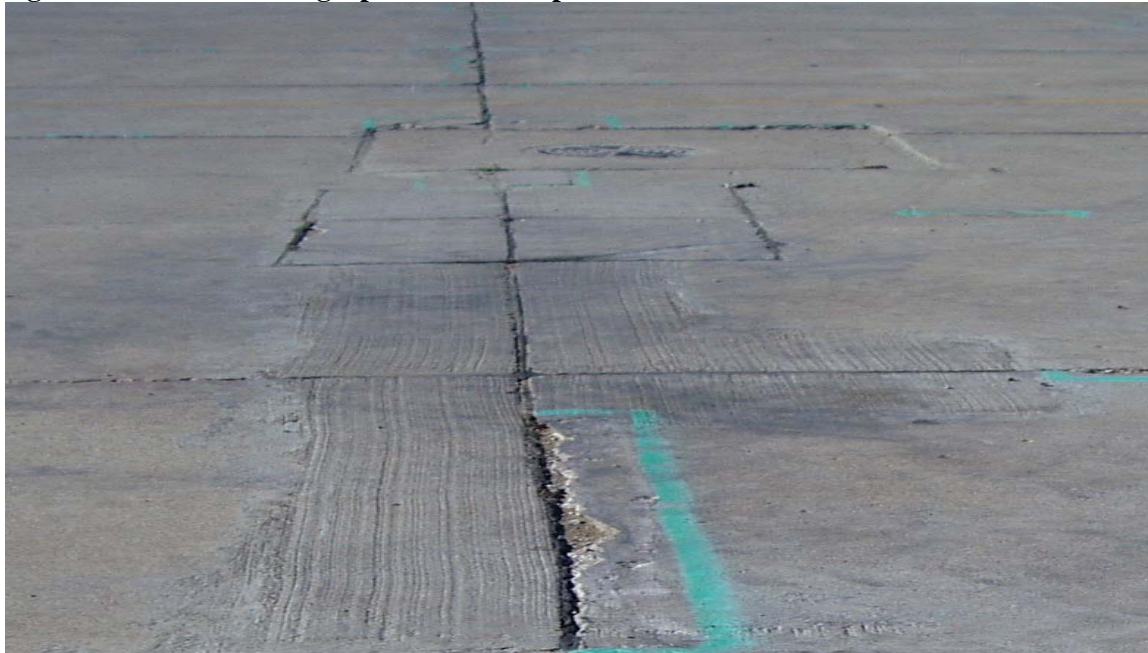
Figure 2. Aircraft Parking Apron Before Repairs
