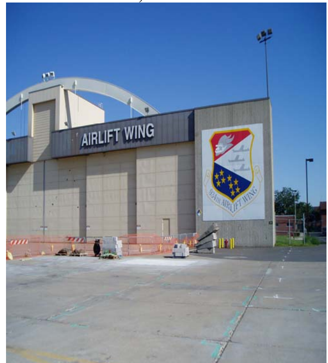
Figure 1. Section of Aircraft Parking Apron Under Repair at the Minneapolis—St. Paul Air Reserve Station, Minnesota
