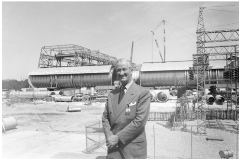
Jack Sverdrup stands in front of PWT during its construction in 1955. An article about PWT in an issue of SPICE, the Sverdrup newsletter, said “When the big wind leaves the nozzle, it rushes into and through the test section which is the heart of the tunnel. It’s a big heart too, for it is 16 feet by 16 feet in cross-section and some 40 more feet long. Here the models or actual aircraft parts and propulsion units will be subjected to the pressure of the transonic or supersonic winds. Here many measurements will be made with a great complexity of instruments.”
