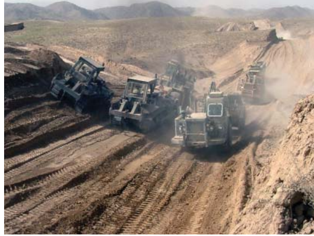
Army engineers from Alaska-based Company C, 864th Engineer Combat Battalion, level a portion of the nearly completed 117-kilometer TK Road, stretching from Kandahar to Tarin Kowt, Afghanistan. (by 1st Lt. Laura Walker)
