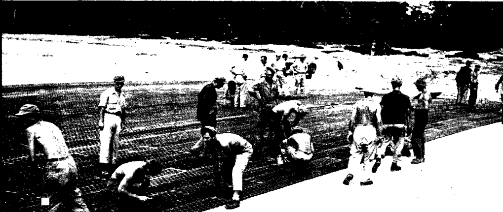
Thirteen days after the 13th ATF had landed, aviation engineers had swept clear the area, bedded it with coral, and had almost completed laying the metal matting, as this photograph shows.
