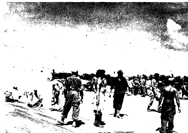
Sunbaked engineers worked furiously to finish the strip in time for the first AAF landings. Photo shows job just about completed.
