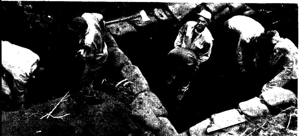
Simultaneously with the establishment of ack-ack emplacements, air raid shelters were set up at regular intervals. Men at right are filling sacks with dirt, lining shelter with them.
