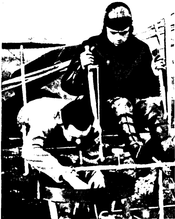
1911. The man fumbling around in this dishpan is Riley Scott who is about to try out his mechanical bombsight. Two 18-lb. bombs hit the target—well, almost anyway.
