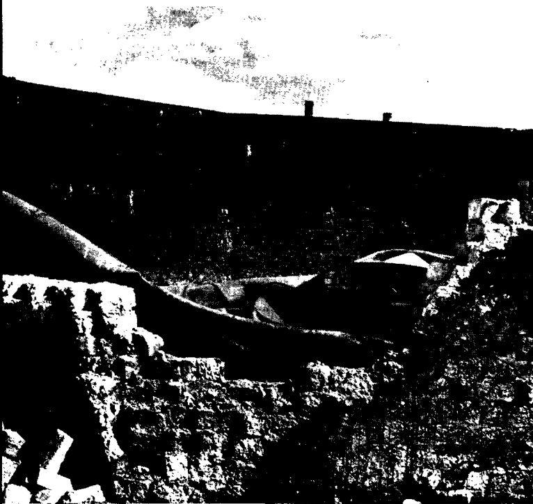
Thick blast walls 20 feet high were reduced to rubble at the Xenia refinery. Oil tank, sheltered by walls, was completely collapsed.
