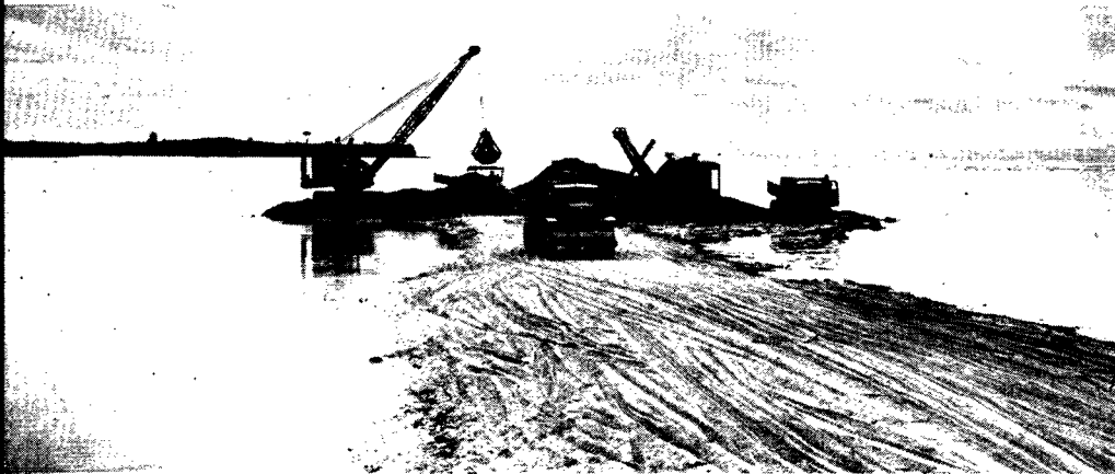
Engineers needed coral to cover sandy loam, which is poor base for steel matting. This reef, extending off Middelburg, furnished all the coral needed, but it could be worked only at low tide.
