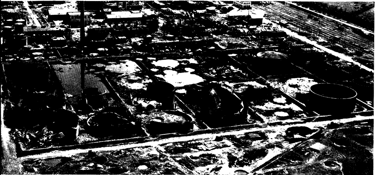
Concordia Vega was virtually demolished by a series of heavy blows during July, 1944. Only two of the tanks in foreground remain intact.
