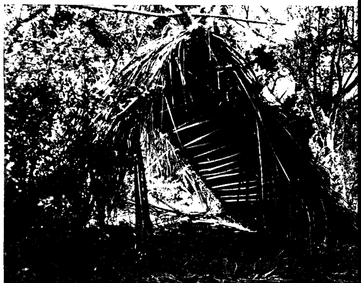
This "A" type lean-to shelter is made of poles bound with palm fibers and covered with mats woven of palm fronds. It is waterproof.
