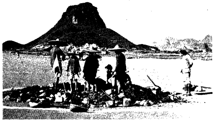
Runway somewhere in China being mined with an ingenious pattern of bombs. Here coolies dig hole at point marked with white circle.
