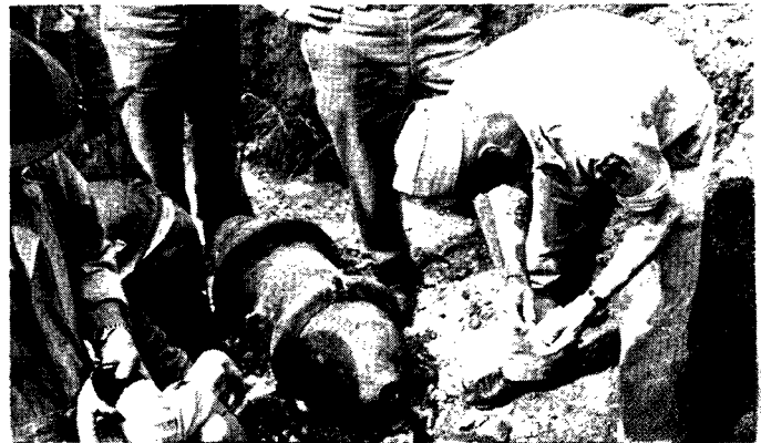
Demolition bomb is placed in hole dug by coolies. Lt. Col. Richard W. Treiber shaves block of TNT which will be put in nose of bomb.
