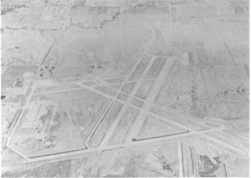
Wichita Municipal Airport, October 1943
