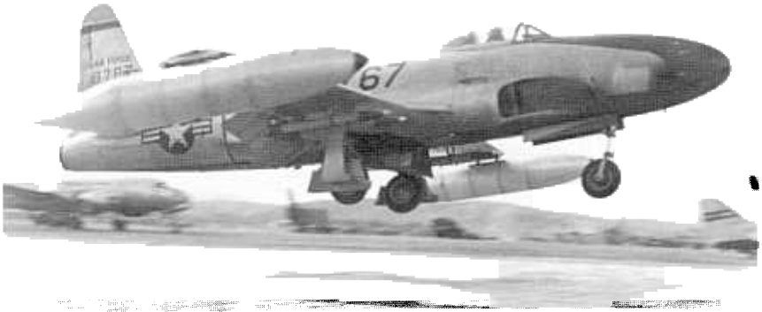
An F-80 Shooting Star takes off for a mission over Korea, December 1950. The enlarged fuel tanks on the wings give the aircraft additional combat range.
